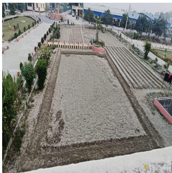
Construction of Poshan Vatika "Ganga Ma Mandal Model" is in progress in KVK, Piprakothi
